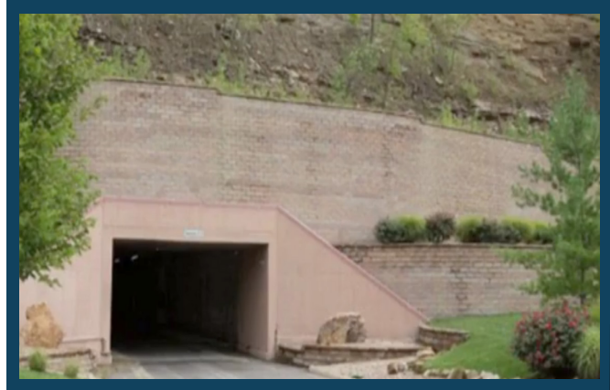
Entrance to Cavern Technologies' 125-foot deep facility
